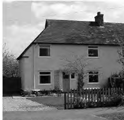
House 513 - Replacement Windows
