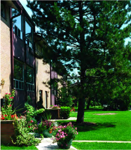
Figure 4: South Hill Village . View of a front façade with exterior storage cabinets for garbage and tools. James Murray and Henry Fliess, Associate Architects, 1954. Photo by Nancy Duff, 1999.
