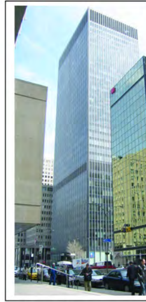
Telus Building Looking South East
