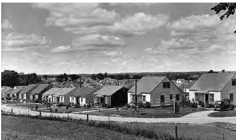
Figure 3: Wartime Houses, Ajax, Circa 1941 Ajax Public Library [P070-000-042]
