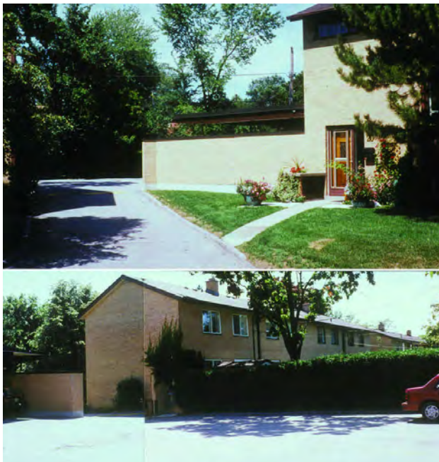
Figure 3: South Hill Village. Views of the parking compound. James Murray and Henry Fliess, Associate Architects, 1954. Photos by Nancy Duff, 1999.
