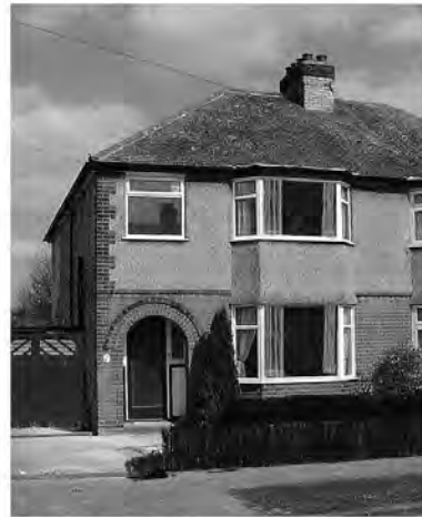
House 517 - Replacement Windows
