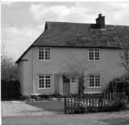
House 512 - Original Windows
