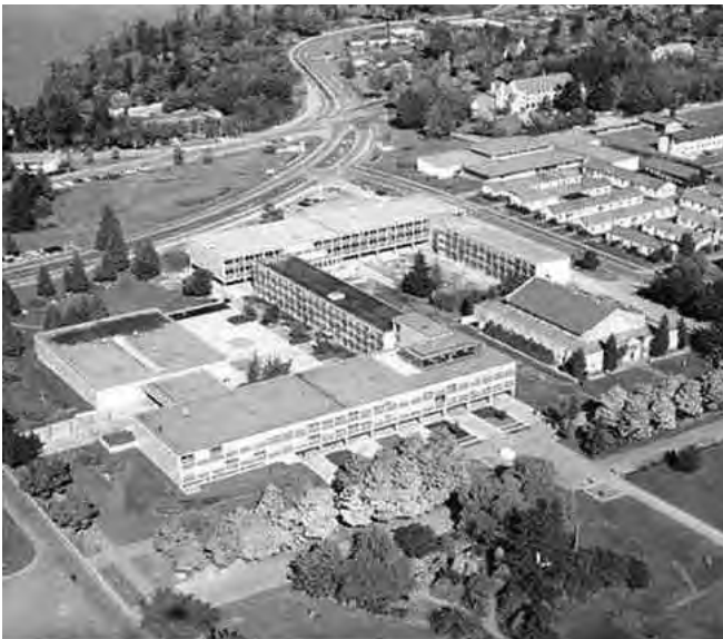
Figure 1: Buchanan Buildings A, B, C, D and E. Aerial photograph looking north-east (1960). Source: UBC Historical Photograph Collection, image # UBC 1.1/2911.
