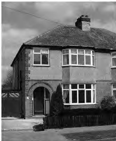
House 516 - Original Windows
