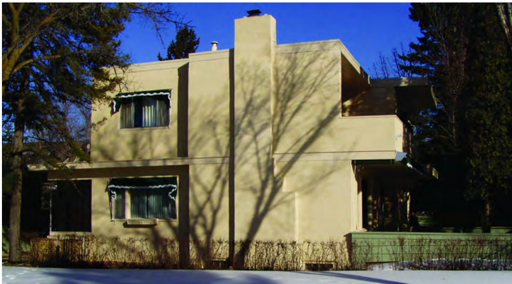
Hyndman Residence, George Heath MacDonald, Architect, 1946-1947 (David Murray Architect)
